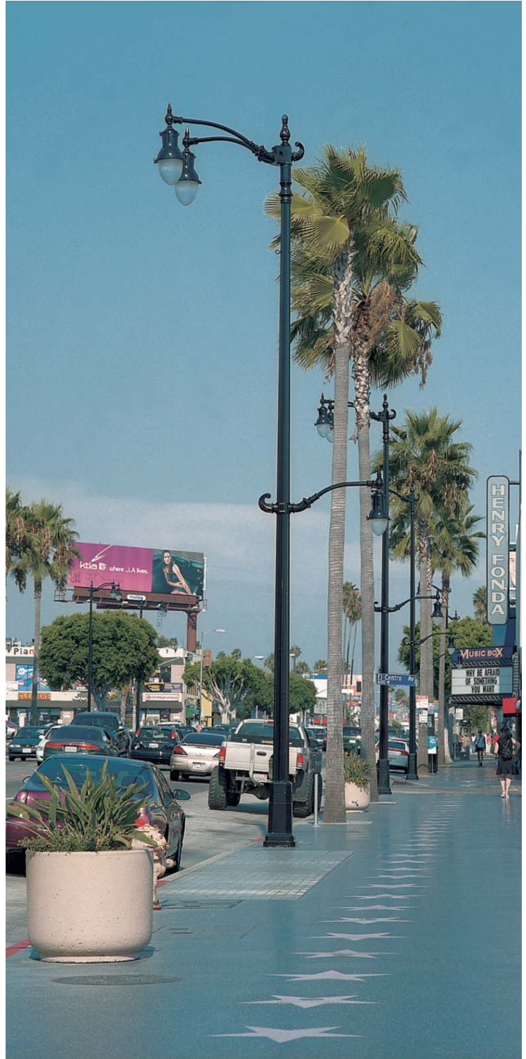
Project: Hollywood Boulevard; Hollywood, California Tear Drop and Pedestrian Tear Drop luminaires on a custom arm and pole
